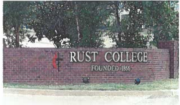
Entrance Wall on Rust Avenue
